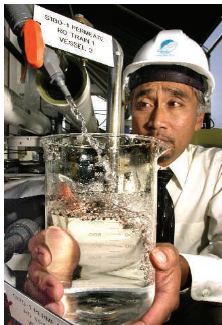
Double duty. A pilot project at a California power plant purifies seawater used for cooling.
